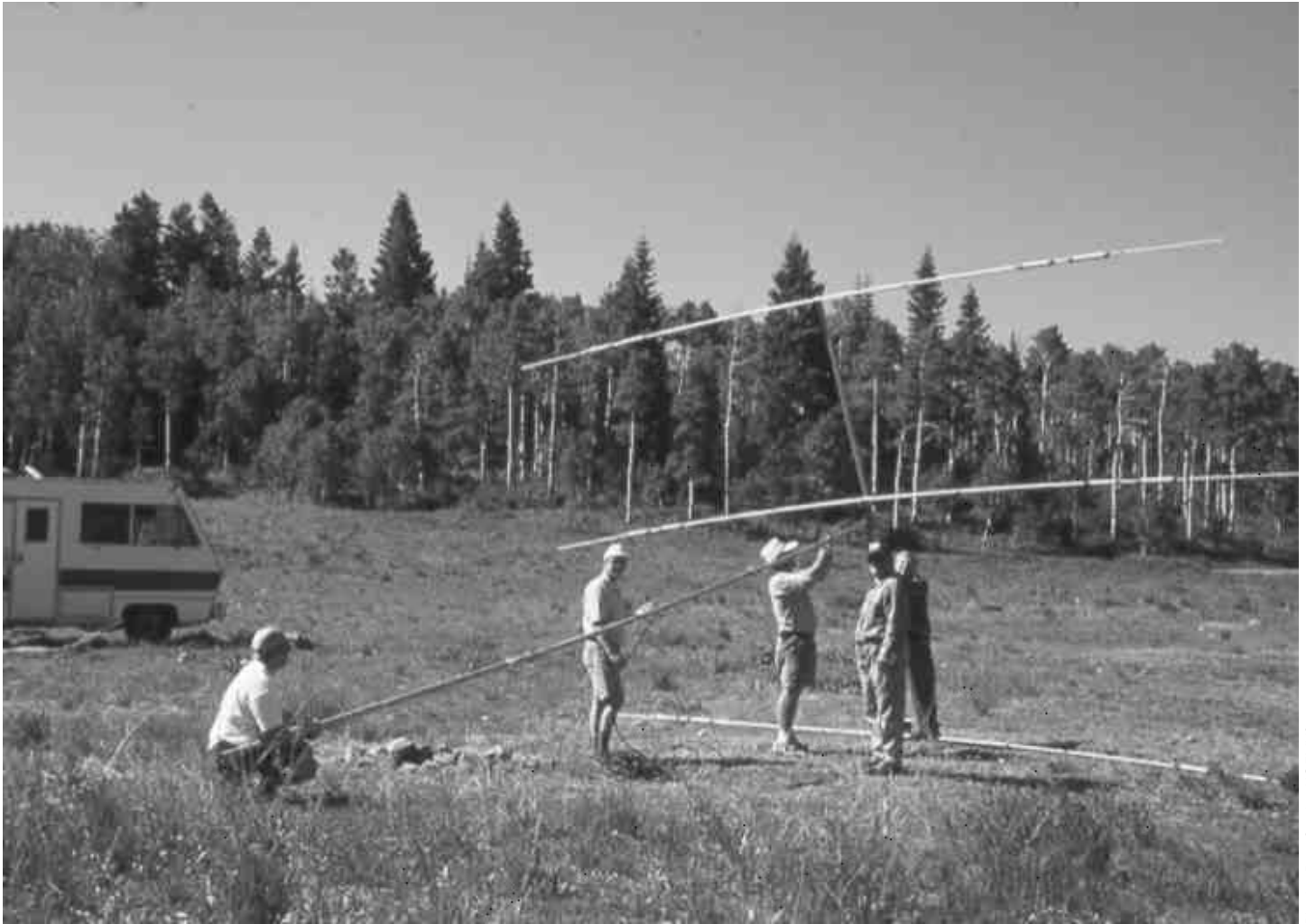
One of the three tri-bander beans is field assembled and raised into position at the UARC Pason Lakes Field Day site.
