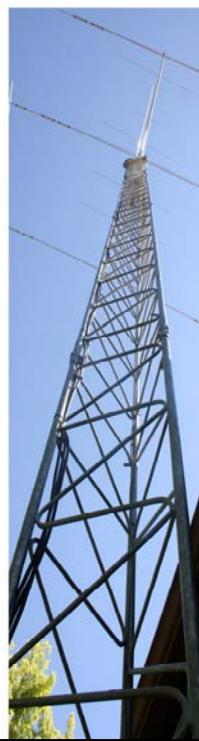
Tower base, 5'. Tower section, 10'. Thrust bearing plate (tower top), Thrust bearing, Yeasu GS-50. Drift pin/ aligning punch = most important tool!
