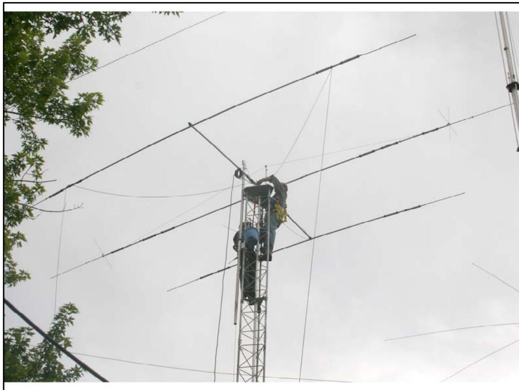
Now the “simple” matter of adding the antennas to the mast, starting with the lowest – and biggest – quad band 3 element beam. Note lines hanging over elements to guide it on the way up. Also note that the coax was attached to the beams when we raised them.
