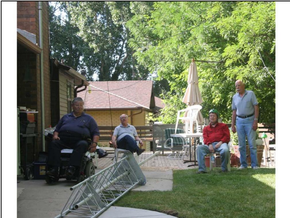
Final section on ground. Note rope to gin pole, rotator base, top plate with thrust bearing, and mast. Can just see other end of rope attached to my chair.
