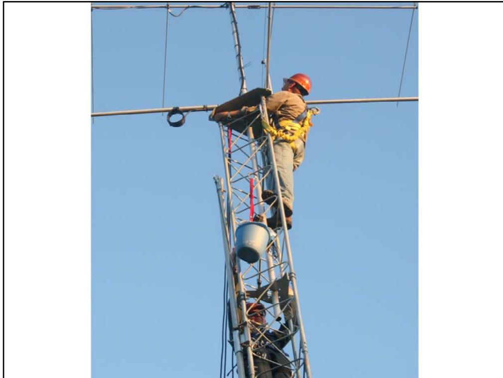
Final steps are to attach coax to mast then push the mast up high enough to mount the rotator, mount it, lower mast into rotator, put bolts in holding rotator on mast, put bolts in attaching rotator to mast. NOTE: rotator does NOT carry weight of mast and antennas, thrust bearing does.
