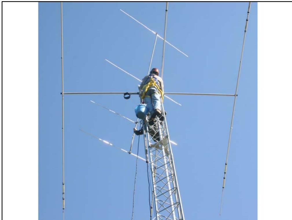
Now thread the 5 element 6 meter beam past the big guy and mount it on the mast.
