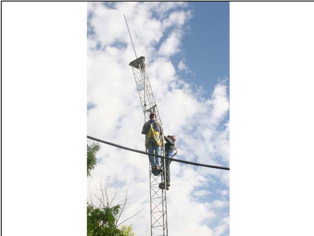
Section is up and at limit of gin pole. LOTS of tension on rope, you can pluck it like a guitar string. Now just a matter of lining up the tower sections.
