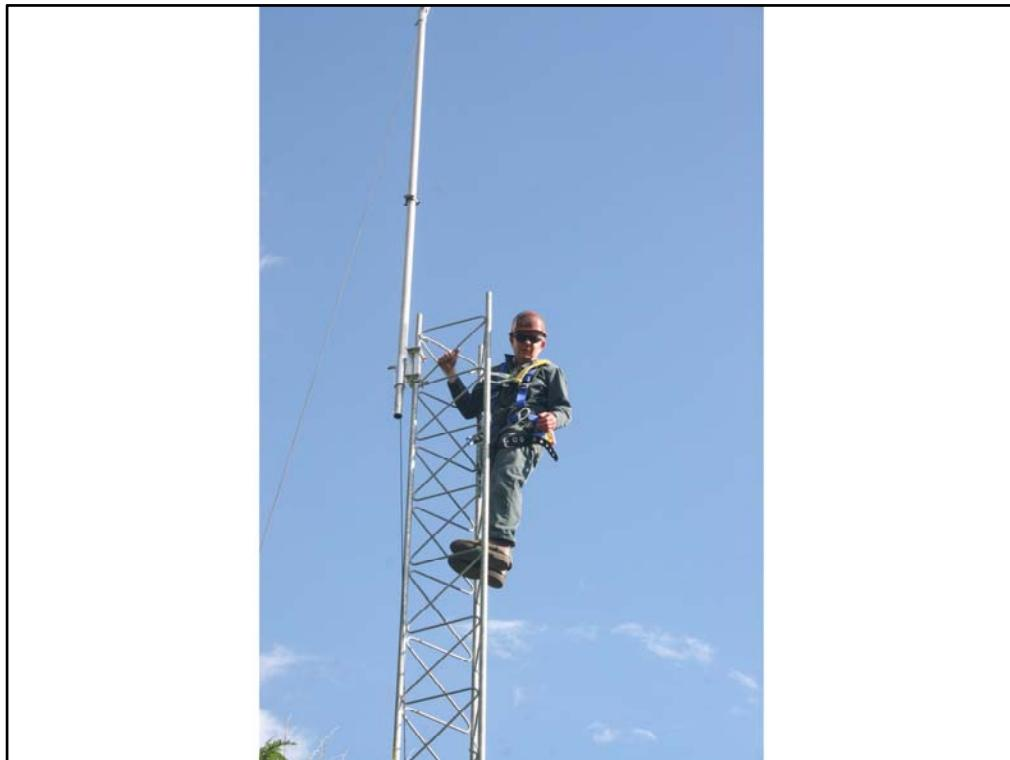
2<sup>nd</sup> and third sections have been erected, now at 30'. Gin pole set up to add final section.
