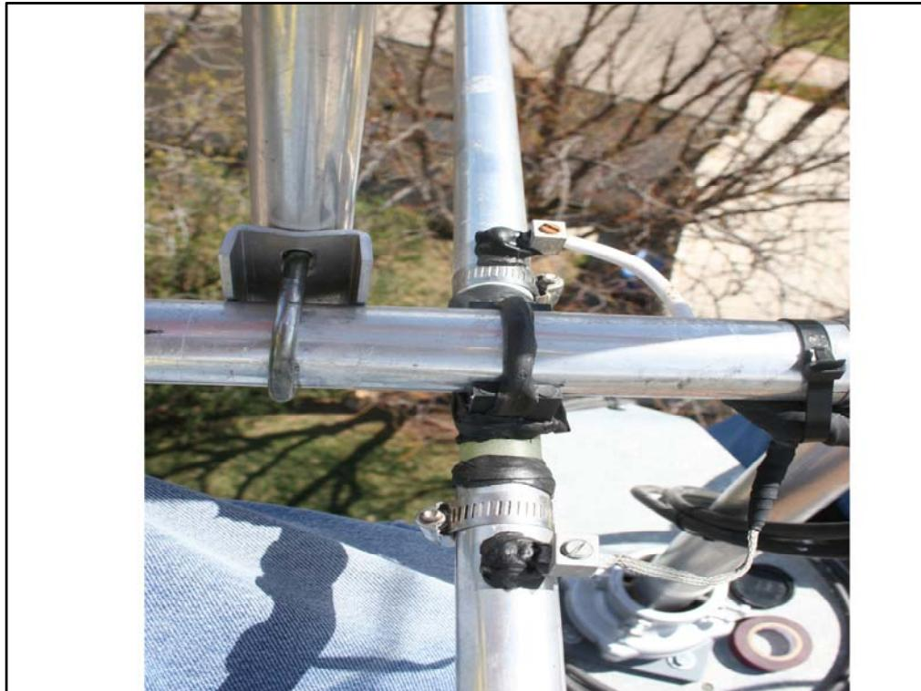
Note how coax is connected and sealed to antenna, thrust bearing, and coax wrap.
