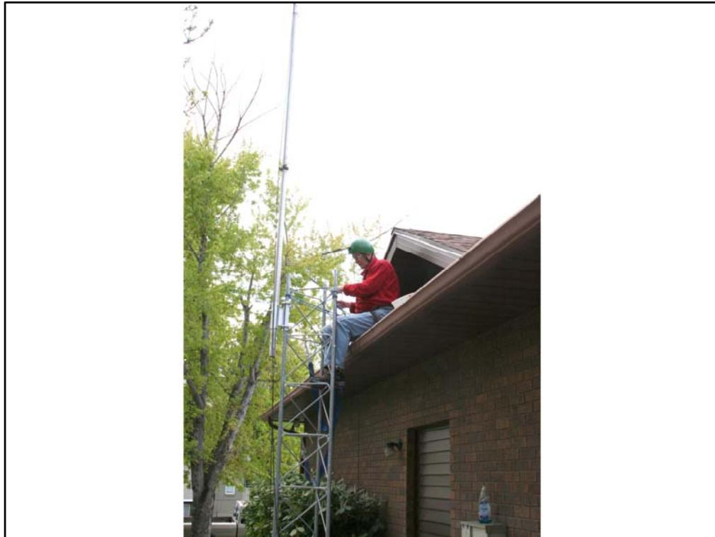
Base is in and first 10' section. Now set up gin pole to add upper tower sections.
