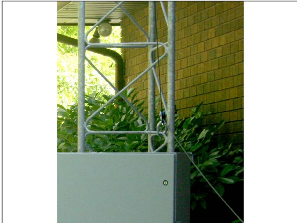
Pulley at bottom of tower – just above NEMA box. Rope goes from piece being lifted up to pulley at top of gin-pole down thru pole to this pulley then to my wheelchair for hoisting.
