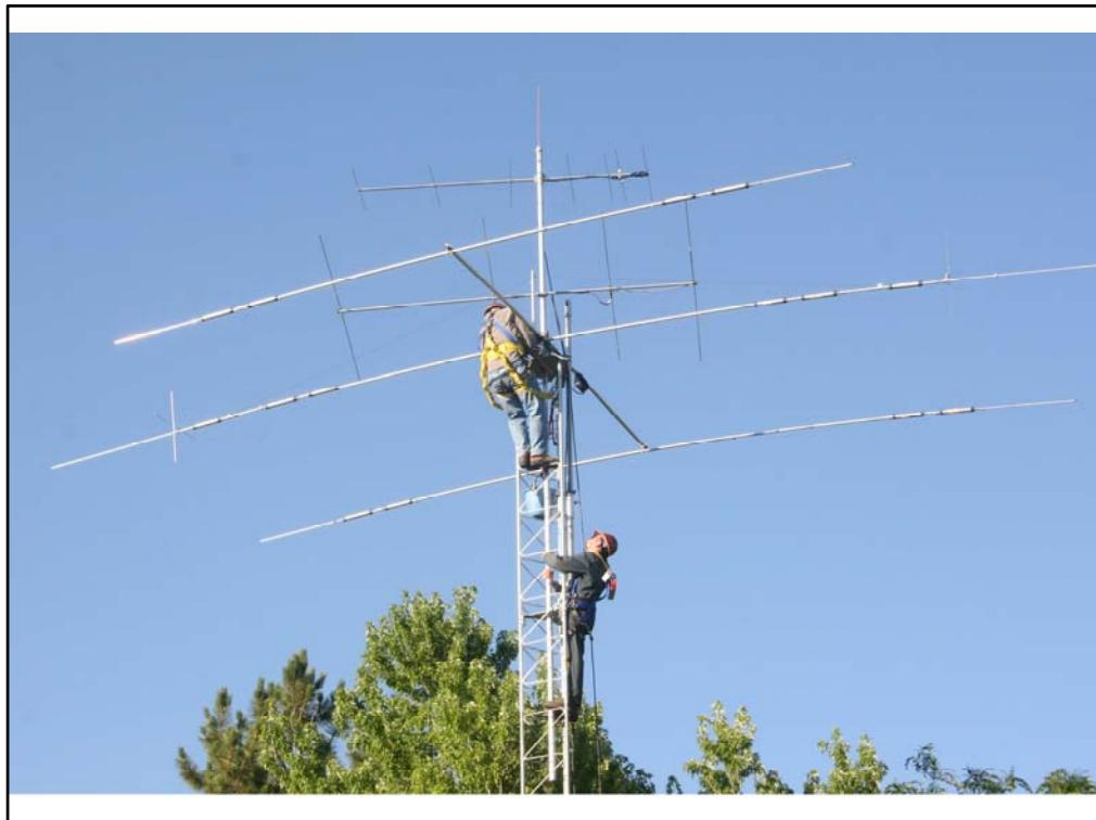
Pat feeds the mast up while John tightens and aligns each antenna with lots of shouting from the ground – very hard for them to hear people on the ground. We marked the mast where we wanted each antenna while the mast was on the ground. Each step involves loosening the thrust bearing while Pat holds the entire weight, pushing the mast up to the next mark, tightening the thrust bearing, then aligning the antenna with the others and tightening it on the mast. Nylox nuts are wonderful!!!!
